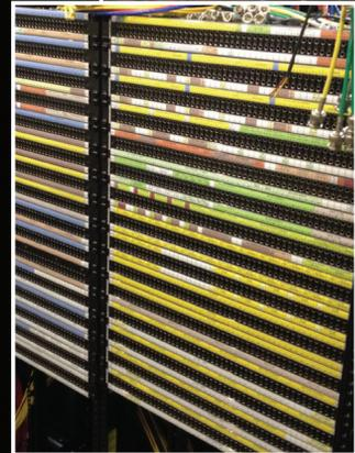
Our VPP (Standard WECO), MVP (Mini WECO) and MMVP (Micro) Video Patchbays are used to patch high definition video in the world's largest broadcast facilities and mobile production units. All of our video patchbay products meet or exceed SMPTE ST 424:2006 specifications. The new MMVP Micro Video Patchbay offers the highest level of density - 96 patchpoints in 1RU!
